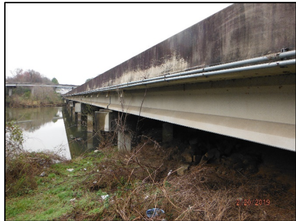
Photo 1 – I-26 Bridge over Saluda River in Richland/Lexington County, SC.
