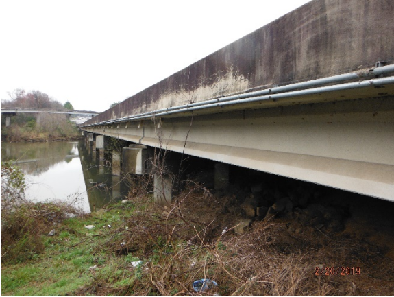
Photo 1. East Side View of Bridge.
