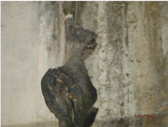
Photo 3. Expansion Joint Board
